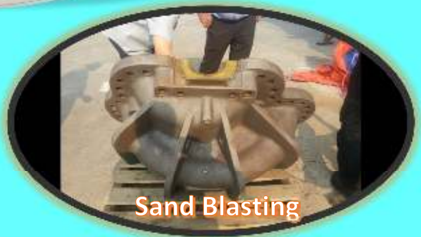
Preparation for Sand Blasting
